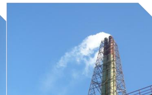
Waste gas – after treatment
